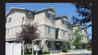
LOGGER CREEK APARTMENTS Boise 112 Units - Sale
